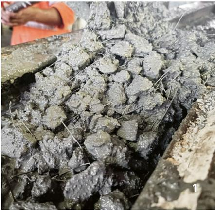
1 Steel Fibre Reinforced Concrete (SFRC)
